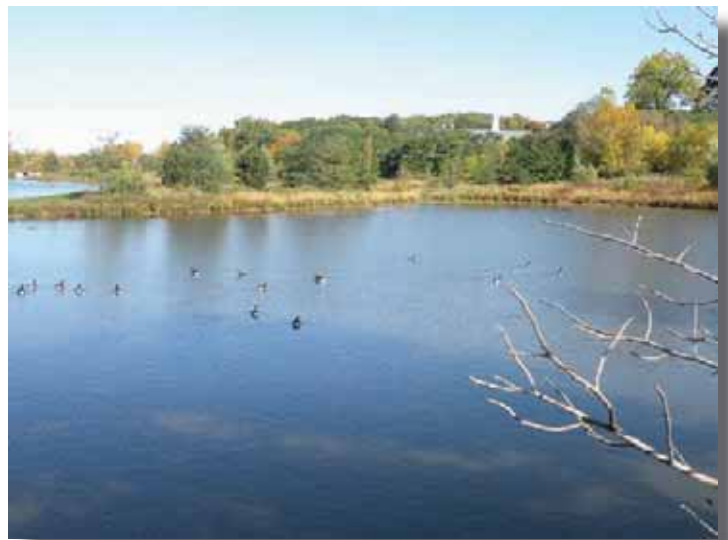
A stormwater pond at King's Bend Park also doubles as a water feature in the park.
